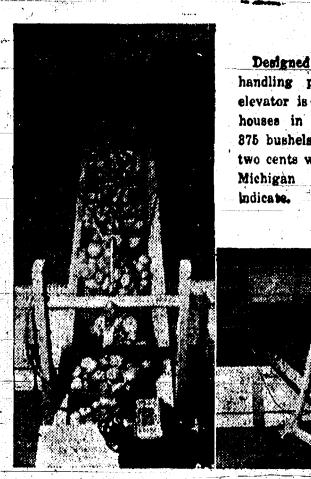
Designed to reduce bruising in handling potatoes, this low-cost elevator is being tried in storage houses in Michigan. It elevates 875 bushels an hour for less than two cents worth of electric energy, Michigan State College tests
